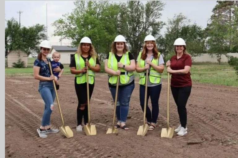
Ground was broken May 16 in Lewis for the foundation of a modular building that will house a pair of new day care centers in the community. Groundbreaking participants, from left, included providers Shana Reed and Yescenia Lopez, Edwards County Daycare Committee member Kelsey Kiewer Holguin, Committee President Trisha Greene, and Committee Secretary Krystle Sandman. Committee members not pictured included Bradley Venters, Schianne Hornbaker, Linette Miller and Karen Myers. Courtesy
